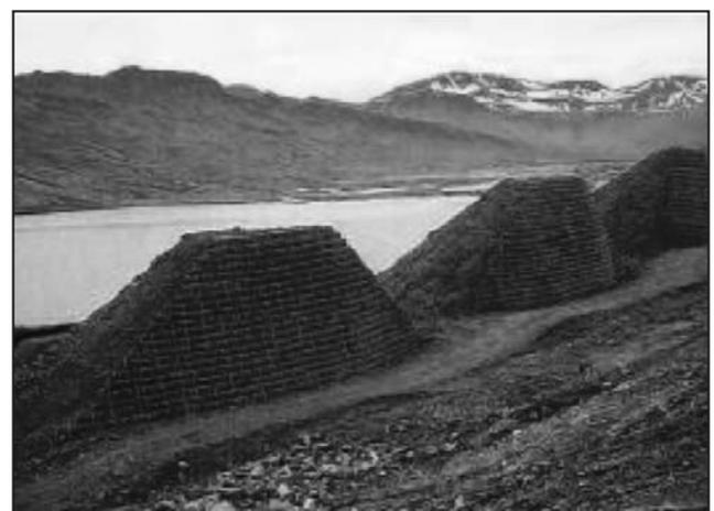
Figure 22. Construction to limit debris flow in Norway
